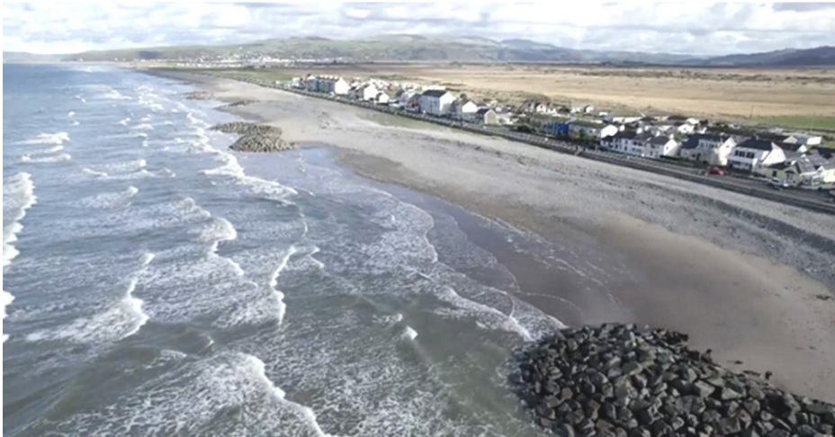
Figure 21. Boulder reefs placed on the beach at Borth.
